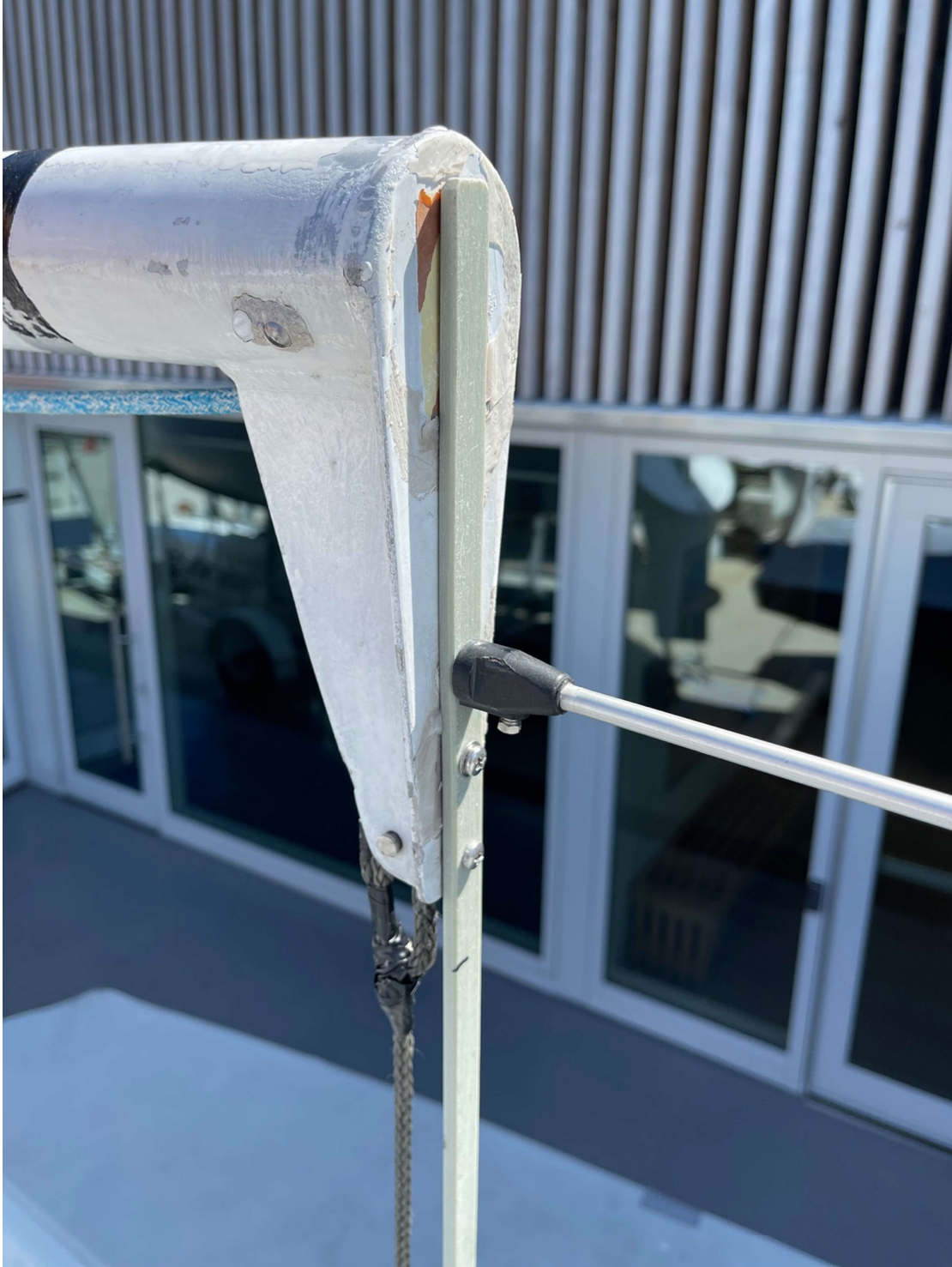
Mast whip bolted/screwed in 3 spots on the mast crane, with the Windex bolt forming one of the attachment points. Tapping screw holes into the aluminum crane can also work, but is more effort and trickier.
